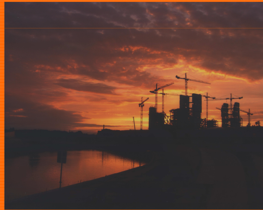
train station (Berlin Hauptbahnhof) under construction
