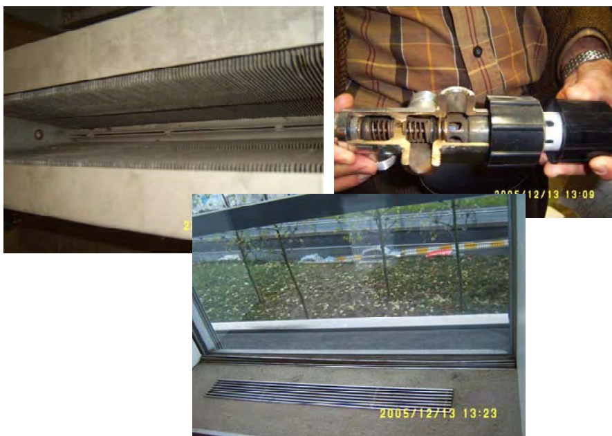
Figure 4: The induction units and their thermostatic valves
