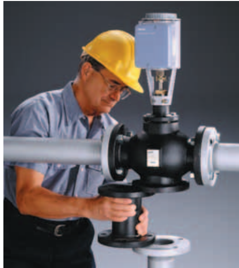
Service flange being removed for service on valve
